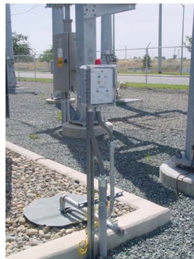
Transformer Oil Containment Installation, Substation: Sacramento, CA
